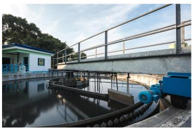
The Tandang Sora STP, which uses an STM-Aerator combining activated sludge and fixed film technology in a compact biological treatment system.
